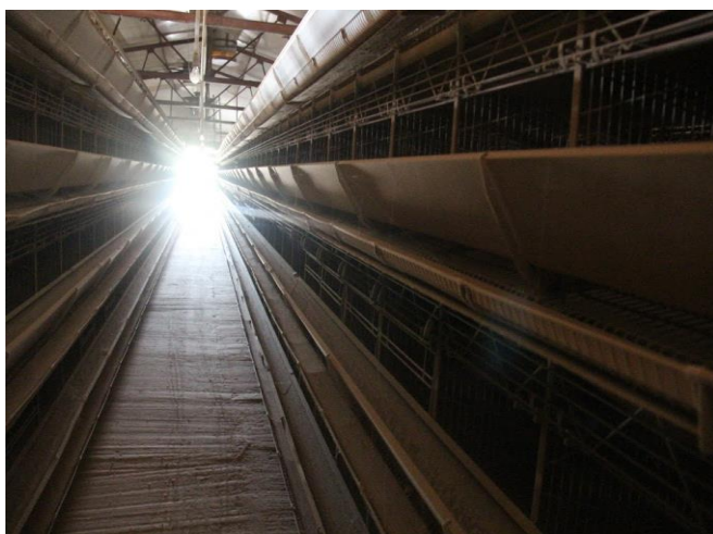
Fig. 5. An example of a prepared facility by combined method, application of the powder and liquid forms of the SiO 2 formulations.
